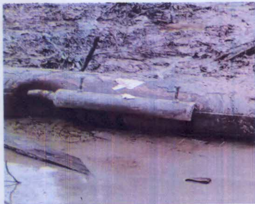
Fig B. SPILL POINT AFTER REPAIR
